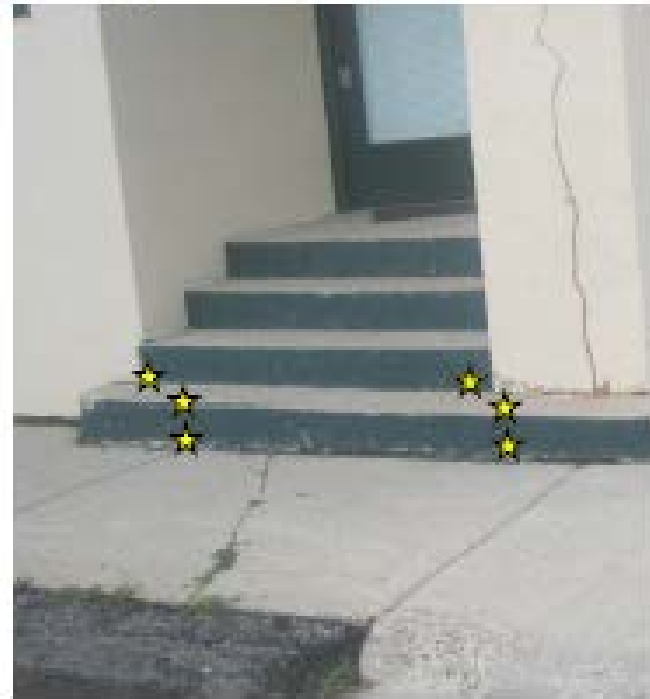
★ Height and tread width of bottom step
