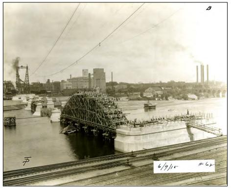
**Figure 11.** June 9, 1915 – Arch falsework, looking northeast (*City of Minneapolis*)
