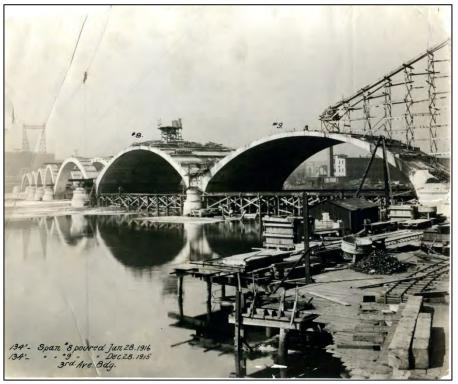
**Figure 15.** c. 1916 – Arch construction, looking west *(City of Minneapolis)*
