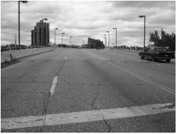
Figure 1. Looking north at the bridge from the south approach. The vehicle barriers are not symmetrical on the south end. A low profile barrier is provided on the east and a taller barrier is provided on the west. The approach roadway pavement is deteriorated and has extensive cracking.
