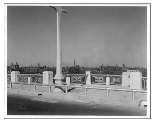
**Figure 24.** 1939 – New sidewalk, railing, and traffic barriers after renovation (*City of Minneapolis*)
