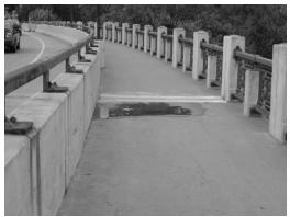
Figure 3. Looking north at the north end of the east sidewalk. Localized ponding adjacent to a reconstructed sidewalk expansion joint is visible. Staining on the vehicle barrier from the metal railing components and anchorages is typical.
