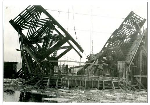
**Figure 12.** c. 1915 – Melan reinforcing for arch ribs (*City of Minneapolis*)
