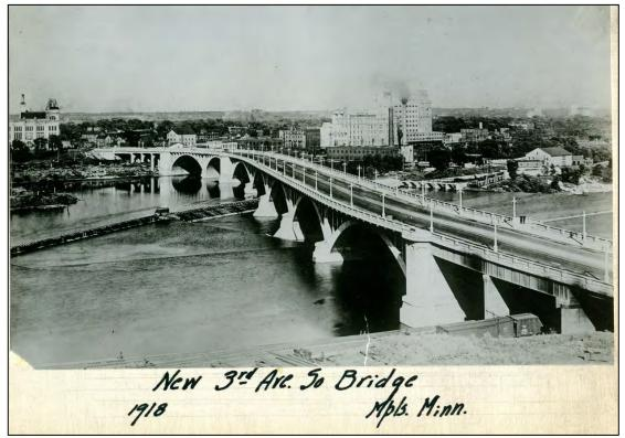
Figure 17. 1918 – Third Avenue Bridge with steel-girder west approach spans in foreground, looking northeast (*City of Minneapolis*)
