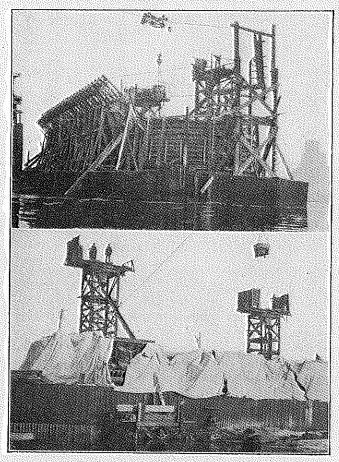
FIG. 6. CONCRETING THE PIERS FOR THE THIRD AVE. BRIDGE
