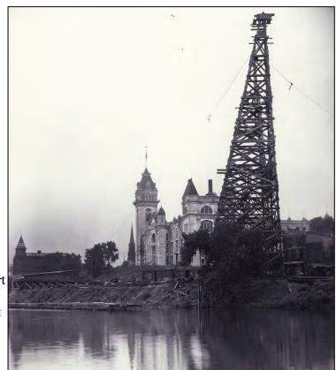
Figure 5. June 29, 1914 – Completed timber tower with part of the concrete plant visible, on the east bank, looking northwest (*City of Minneapolis*)
