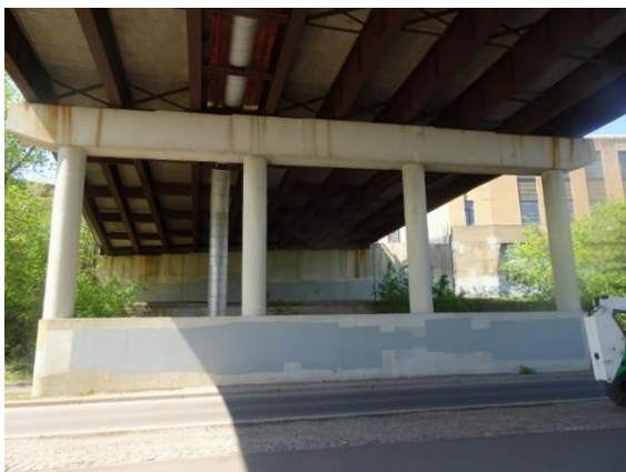
Figure 2.29. South approach framing, looking toward Bent Pier 1 and south abutment.
