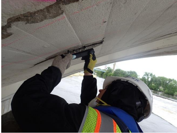
Figure 3.7. Resistivity survey with Resipod (arch rib underside).
