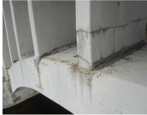
b) 3rd Avenue Bridge (2017).
