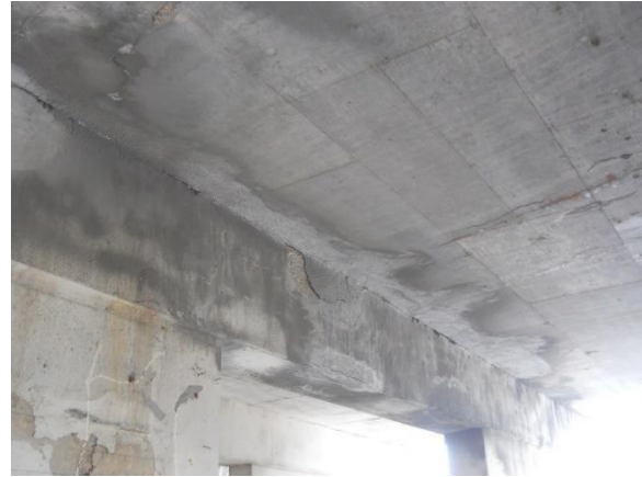
Figure 4.15. Slab underside concrete repair at expansion joints.
