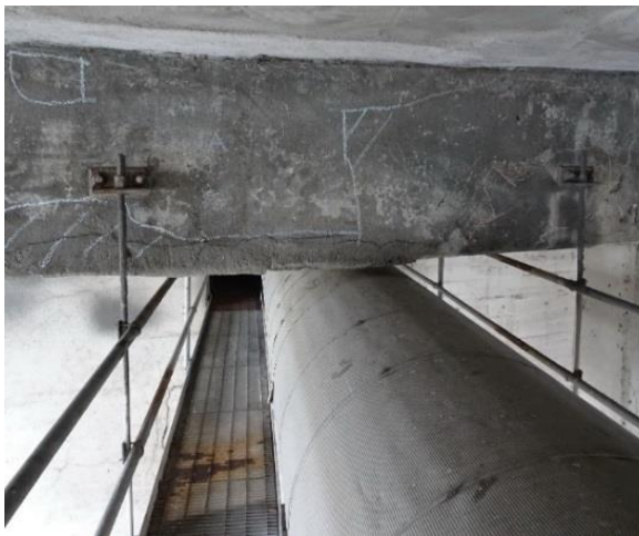
Figure 2.35. View of catwalk and water main suspended from cap beam.
