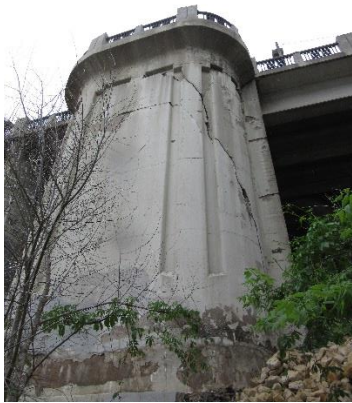
Figure 5.18. Pier 8, downstream face.
