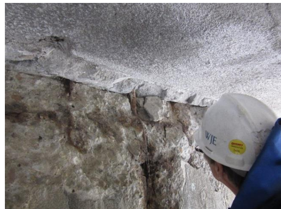
Figure 5.34. Close-up of vertical dowels, showing repair concrete tight against dowels.
