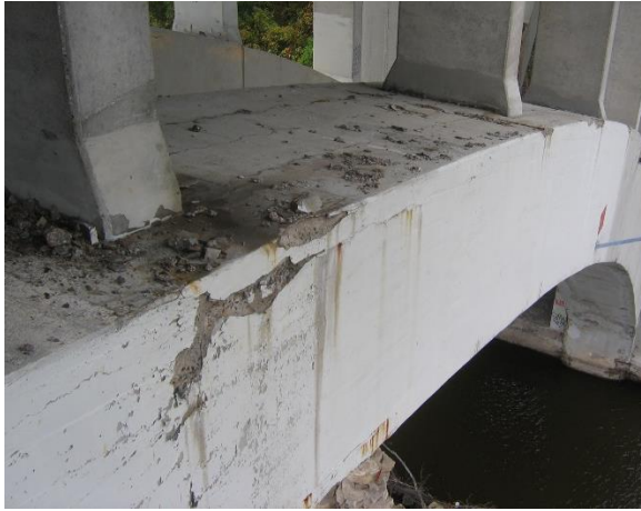
a) Franklin Avenue Bridge (2008).
