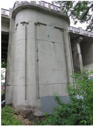
Figure 5.22. Pier 8, upstream face.
