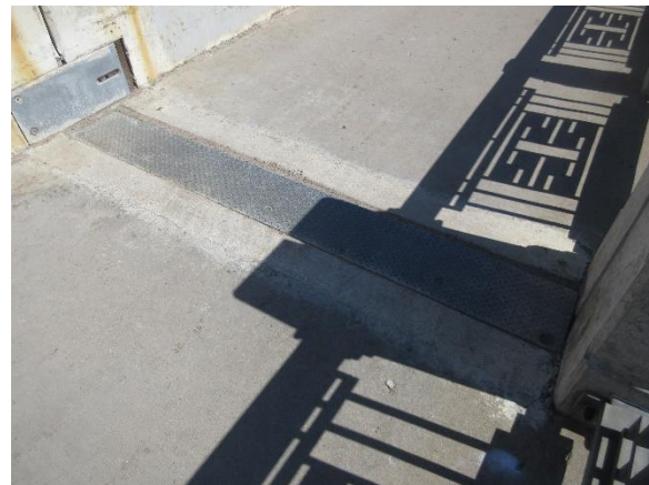
Figure 4.28. Repair material at steel cover plates over strip seal joints.
