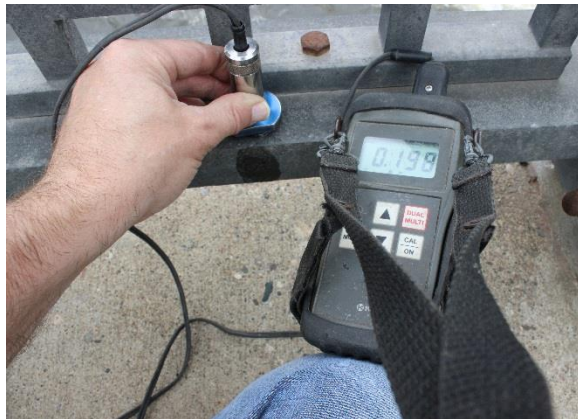
Figure 3.16. Ultrasonic thickness measurement on aluminum railing.
