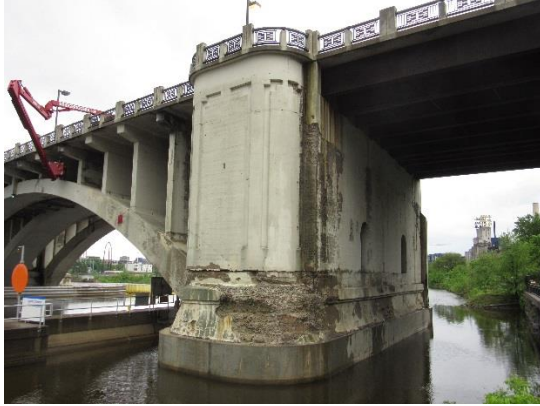
Figure 2.21. Overall view of Arch Pier 1 from upstream side.
