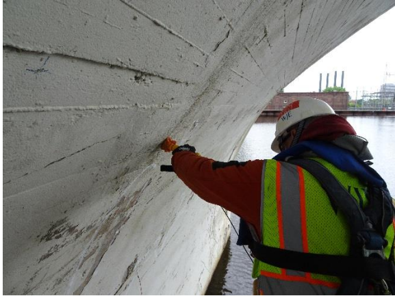
Figure 3.5. HCP survey with CSE electrode and volt meter (barrel arch underside).
