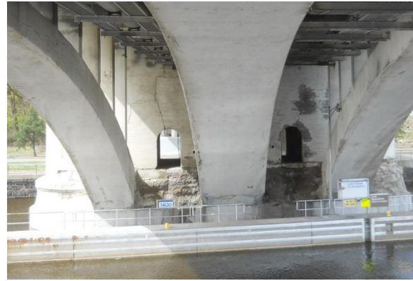
Figure 2.22. Arched openings in the walls of Arch Pier 1.
