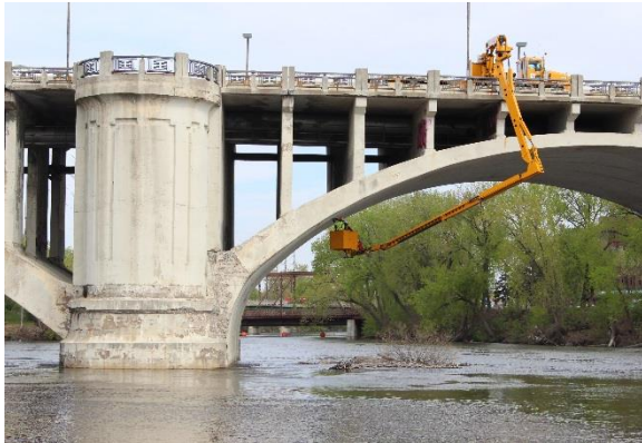
Figure 2.23. Overall view of Arch Pier 6 from downstream side.
