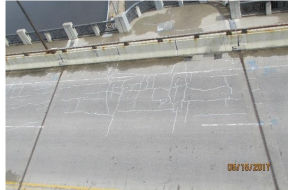
Figure 5.9. Photograph at pier showing strip seals and extending through roadway and sidewalk.
