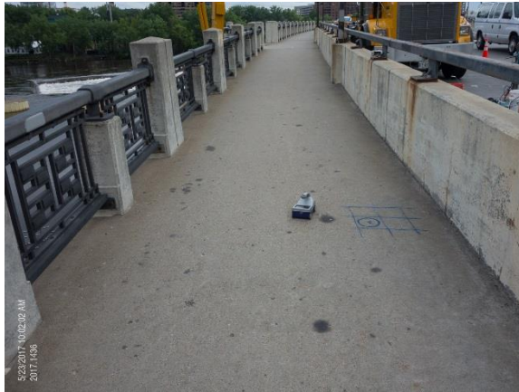
Figure 4.79. Overall view of sidewalk on approach.
