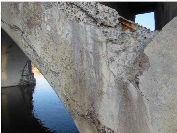
Figure 4.62. Exposed Melan truss angle at barrel arch.
