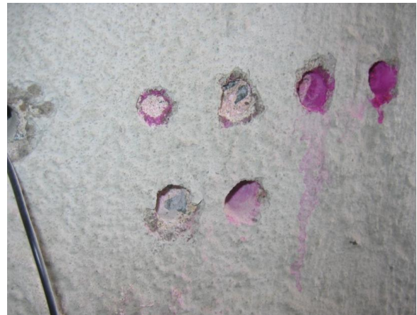
Figure 3.15. Example of incremental drilling to determine depth of carbonation.
