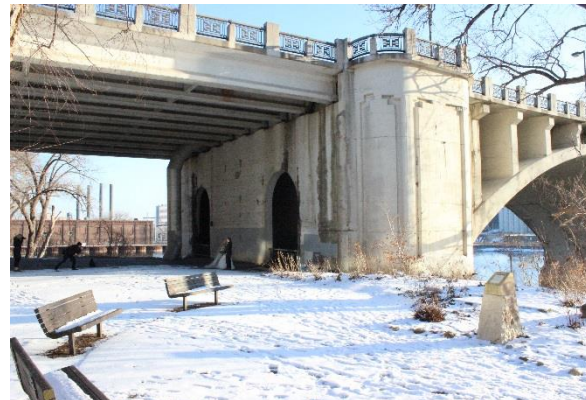
Figure 2.28. Arch Pier 8, upstream side
