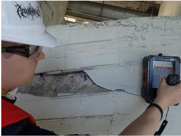
Figure 3.12. GPR survey on arch rib face
