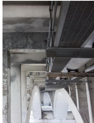
Figure 2.36. Catwalk and water main spanning parallel to arch ribs.
