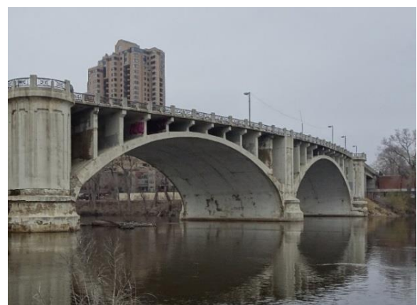
Figure 2.18. Typical view of barrel arches in Arch Spans 6 and 7.
