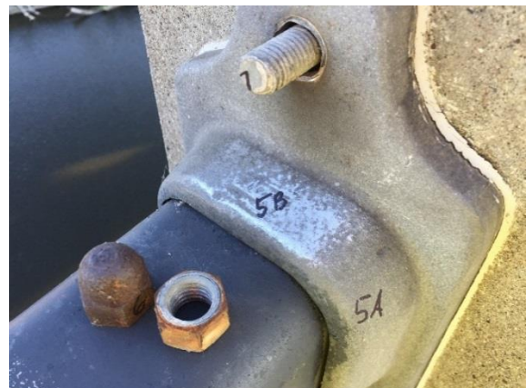
Figure 3.21. Disassembly of railing connection for XRF testing of various components.
