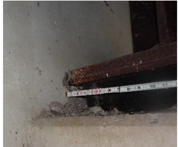
Figure 4.84. Pier 1 expansion bearing near-restricted movement between steel girder and pier wall.
