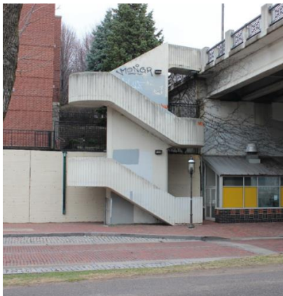
Figure 2.31. Spiral stairway at northwest corner of north approach.
