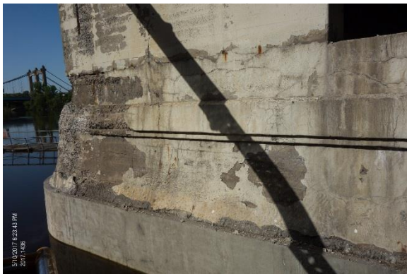
Figure 4.75. Concrete jacket at the base of Pier 1.
