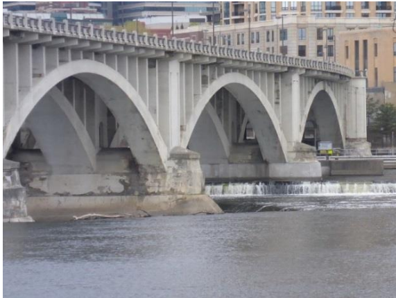
Figure 2.15. Overall view of arch ribs supporting spandrel columns and cap beams.
