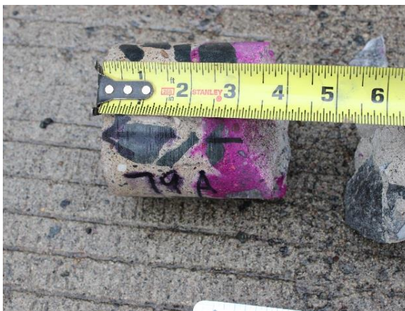
Figure 3.14. Example of field carbonation measurement.
