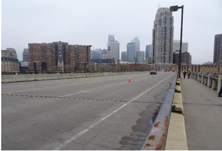
Figure 2.11. Overall photo of existing bridge deck.
