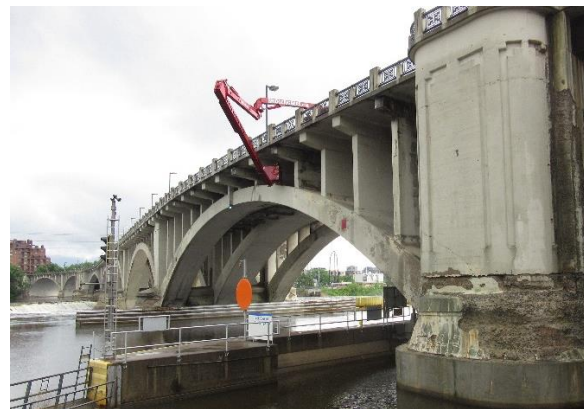
Figure 2.3. Overview of the bridge from the south bank (upstream side).
