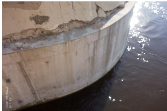
Figure 4.76. Concrete jacket at the base of Pier 2.
