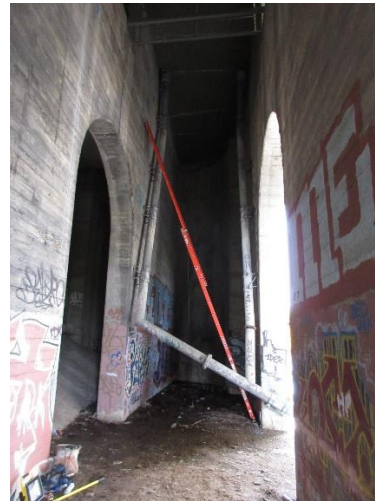
Figure 2.24. Interior of Pier 6.
