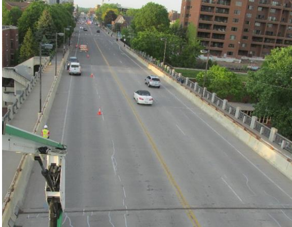
Figure 2.37. Overview of north approach from bridge.
