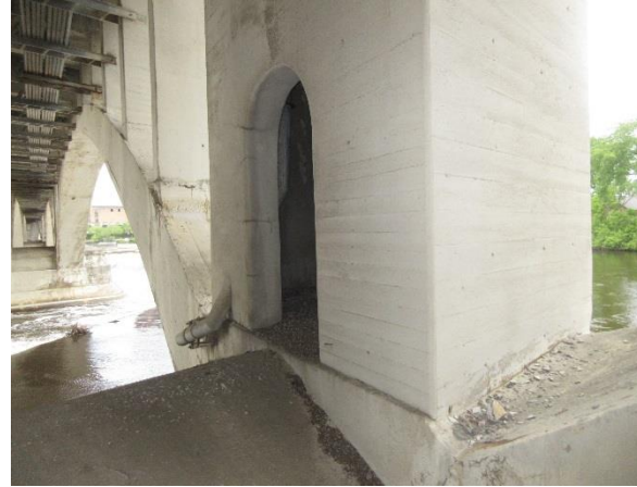
Figure 2.26. Typical pier column (Pier 2 shown).
