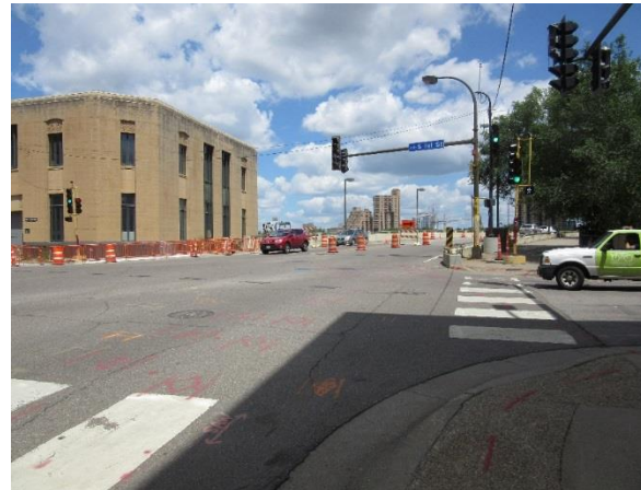
Figure 2.38. Overview of south approach to bridge.
