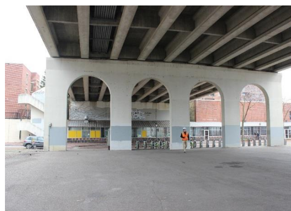
Figure 2.30. North approach framing, looking toward Bent Pier 2 and north abutment.
