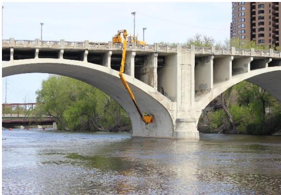
Figure 2.27. Arch Pier 7, downstream side.
