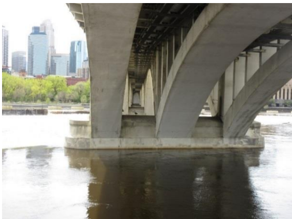
Figure 2.17. Typical view looking along the arch ribs from beneath Arch Span 5.
