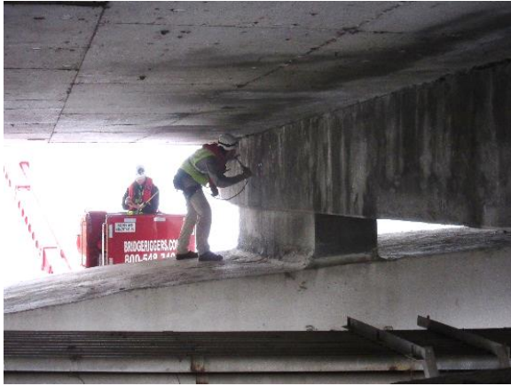
Figure 2.12. Typical spandrel column and cap beam, supported on arch rib.
