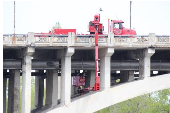
Figure 2.13. Typical spandrel columns and cap beams, supported on arch rib.
