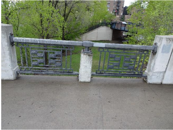
Figure 4.99. View of typical pedestrian railing panel.
