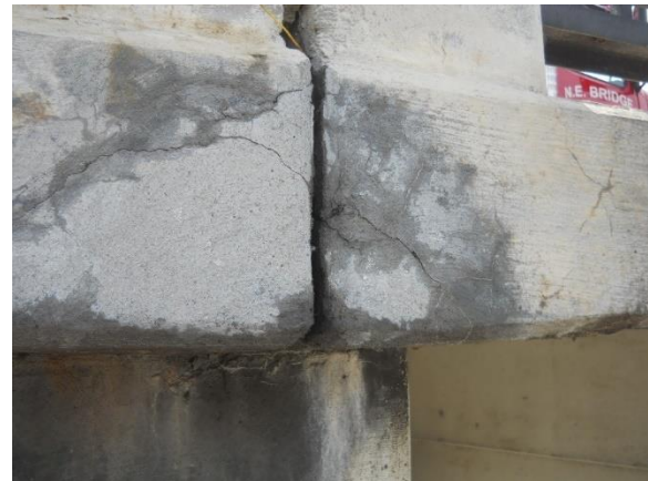
Figure 4.13. Upstream deck edge repair at expansion joint.
