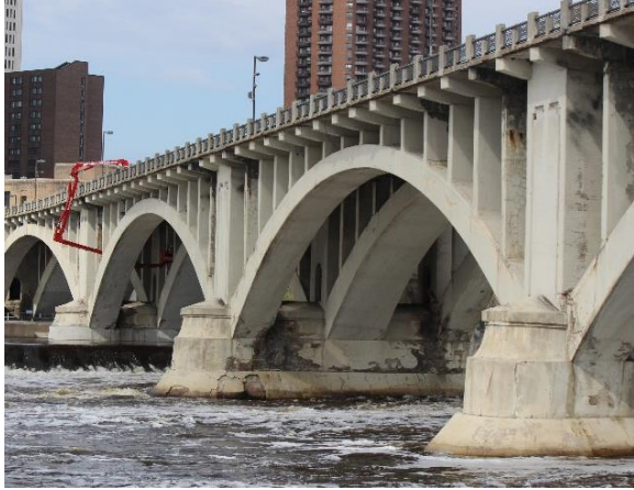
Figure 2.25. Typical view of piers with three pier columns (Piers 2, 3 and 4 shown).
