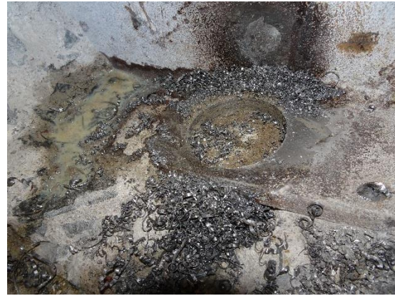
Figure 3.4. Melan truss steel sample removed by coring.
