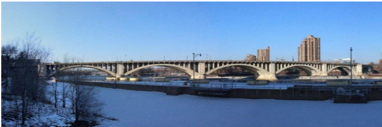
Figure 2.1. Overview of the bridge from the downstream side, south bank.
