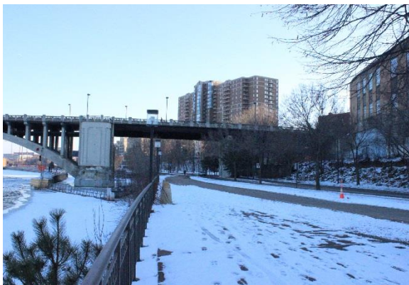
Figure 2.39. View looking east along West River Parking below south approach.
