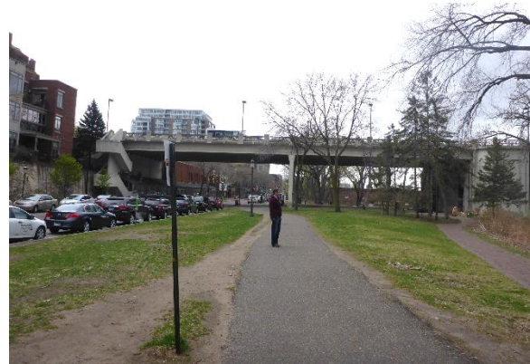
Figure 2.40. View looking east along Main Street below north approach.
