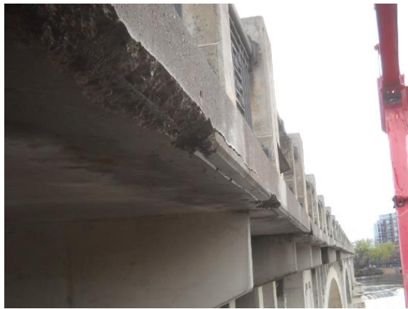
Figure 4.10. Downstream deck edge condition.
