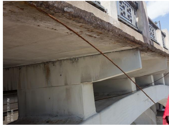
b) 3rd Avenue Bridge (2017)
