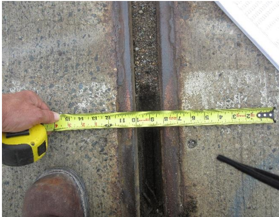
Figure 5.15. Original gap measurements using tape measure at shoulder stripe.
