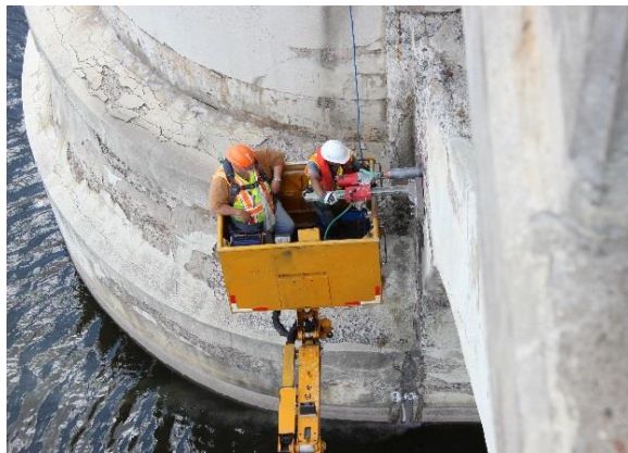
Figure 3.1. Example of concrete core removal.
