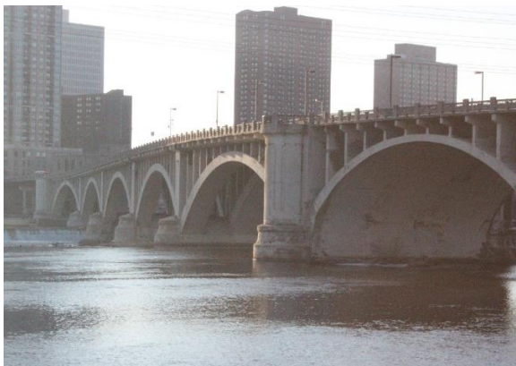
Figure 2.2. Overview of the bridge from the north bank (downstream side).
