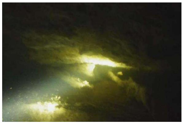
Photo 15 - View of Undermined (Undercutting) cavity at Pier 5, Looking South
