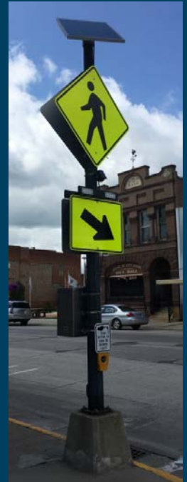
Push button and motion activated, LED-enhanced crossing system in Sleepy Eye, MN (1 st Ave / HWY 14)
