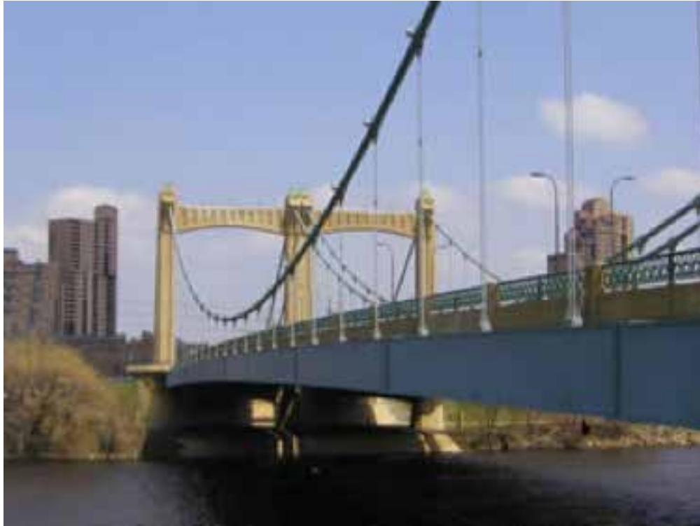
Suspension bridge in Minneapolis, Minn. Photo credit: Minnesota Department of Transportation
