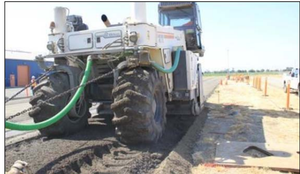
Figure 3.5: FDR-NS: Test track recycling.
