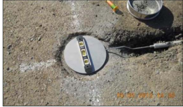
Figure 4.4: Pressure cell installation.
