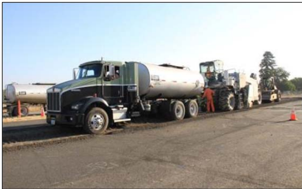
Figure 3.14: FDR-EE: Recycling train.
