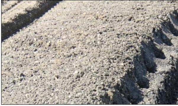
Figure 3.8: FDR-NS: Pulverized material.
