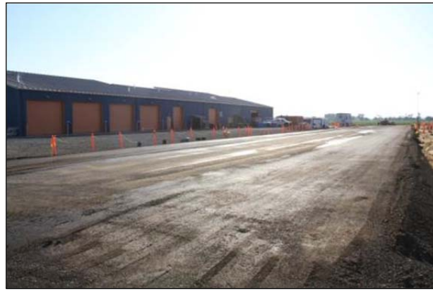
Figure 3.11: FDR-NS: Surface leveling with a grader.
