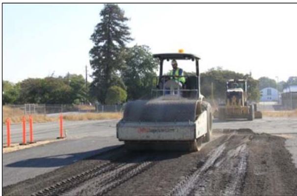
Figure 3.18: FDR-EE: Excess fluid during and after compaction with smooth drum roller.
