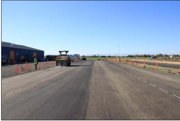
Figure 3.38: First lift of asphalt concrete after compaction.
