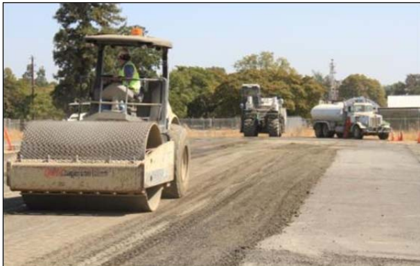
Figure 3.10: FDR-NS: Compaction with smooth drum roller.
