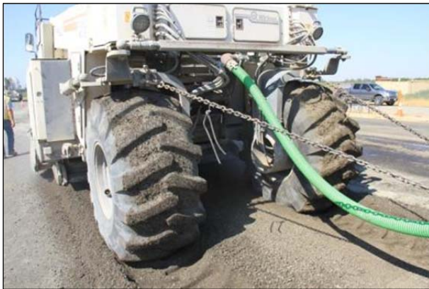
Figure 3.23: FDR-FA: Uniform mix behind recycler.
