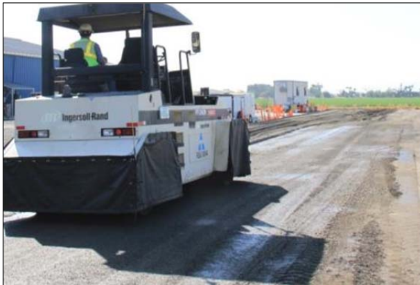
Figure 3.12: FDR-NS: Compaction with rubber-tired roller.
