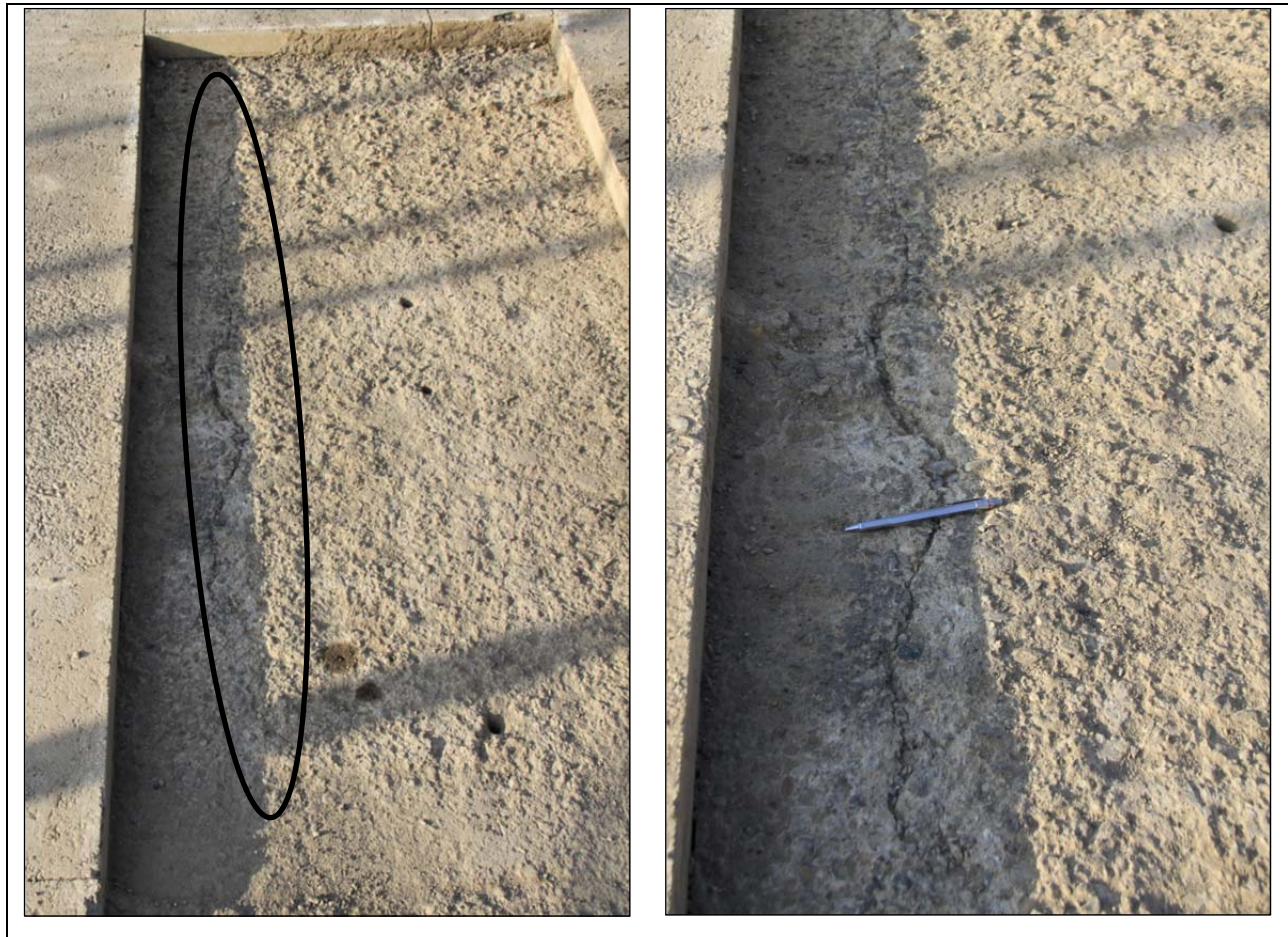
Figure 8.11: 682HB: Test pit photographs.
