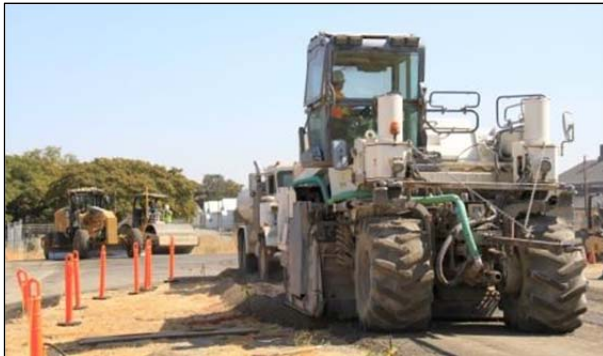
Figure 3.5: FDR-NS: Test track recycling.
