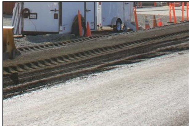
Figure 3.32: FDR-PC: Uniform mix after second recycling pass.
